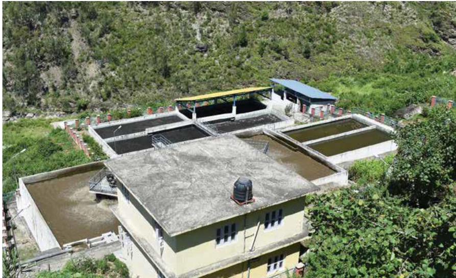
Figure 10 Sewage Treatment plant at Village Jhakri
